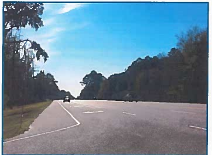
Streetscape: Southwest view of State Route 170
