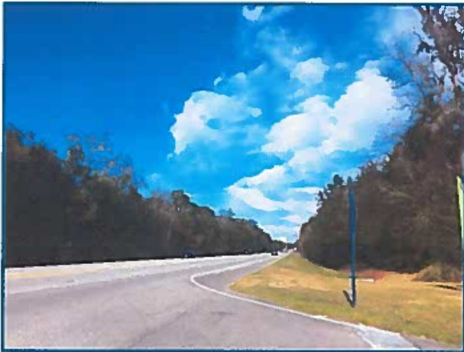
Streetscape: Northeast view of State Route 170
